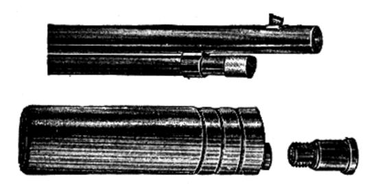
Through the silencer, lengthwise, there is a clear passage for the bullet and surrounding the passage are laminæ for whirling and retarding the powder gas. In its present form it is a sort of necessary evil: a crude protuberance performing an incomplete function. The interested rifleman may yet simplify and improve it, thereby conferring a benefit and receiving, perhaps, a fortune.
